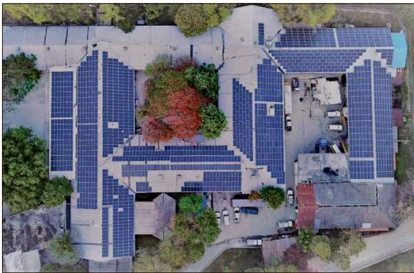
Andrez solar segls tetgs digl HAS suainter ca Christian Hassler, Christoph Baumann a lur squadra vevan instalo 1200 m 2 panels.
